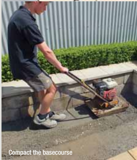
Excavate the area then fill with basecourse
