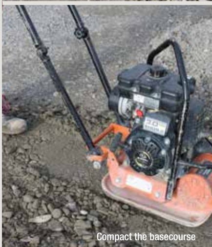
Excavate the area then fill with basecourse
